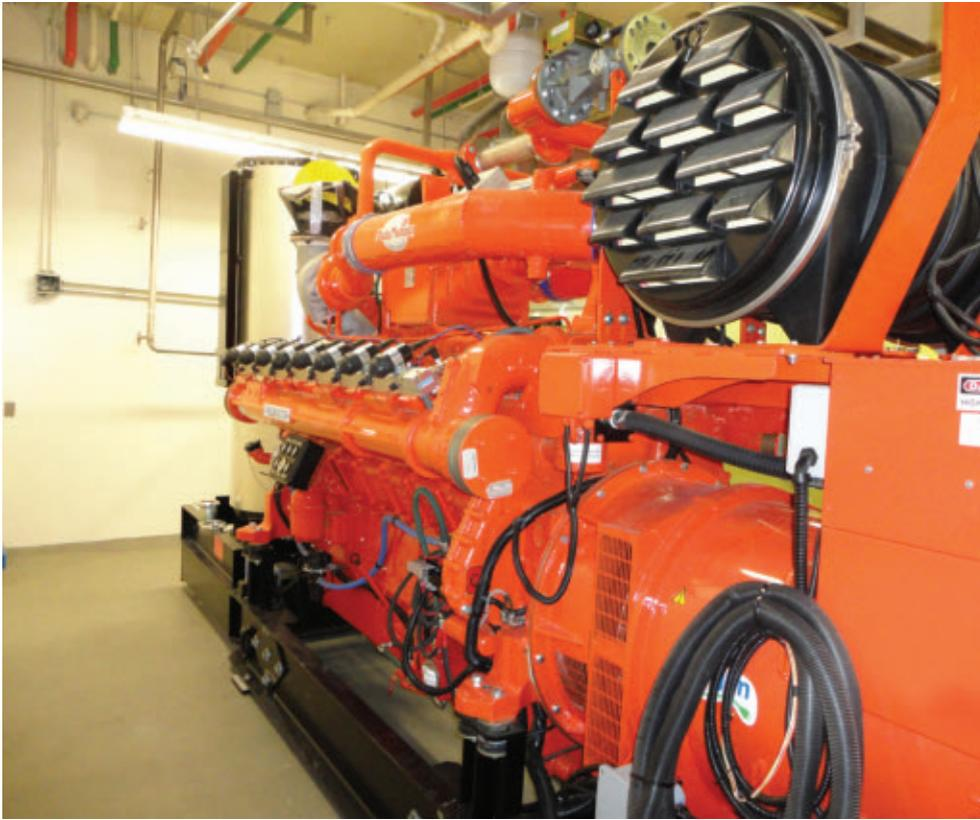
The New Belgium brewery uses a 500 kWh Guascor biogas engine in a CHP application, located in an engine room next to the brewhouse.
