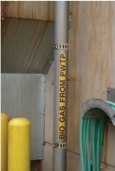
Biogas is piped from the gas balloons near the company's dedicated process water treatment plant (PWTP) into the engine room.
