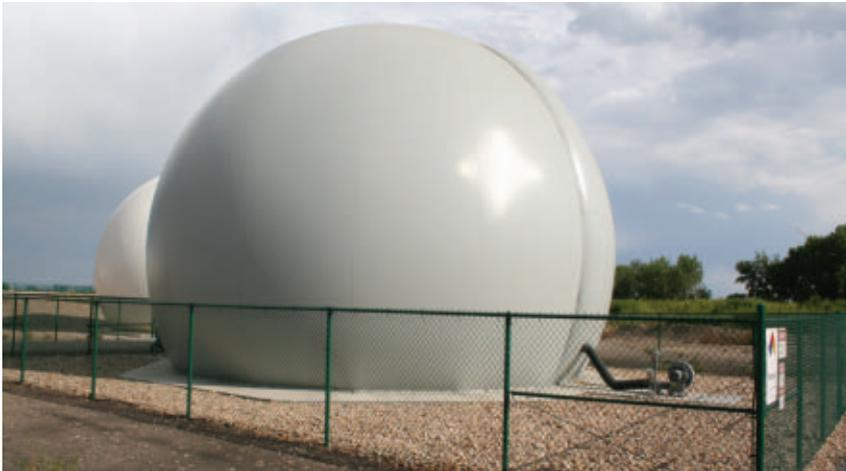
Biogas is stored in two large balloons near the water treatment plant. The outer layer is a hard shell, while inside a blower ensures that positive pressure is maintained between the shell and an interior membrane. When the methane is being used, the pressure collapses the balloon and pushes the methane out.
