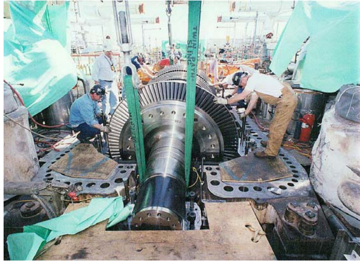
Figure 7 – HPT Installation at Salem
