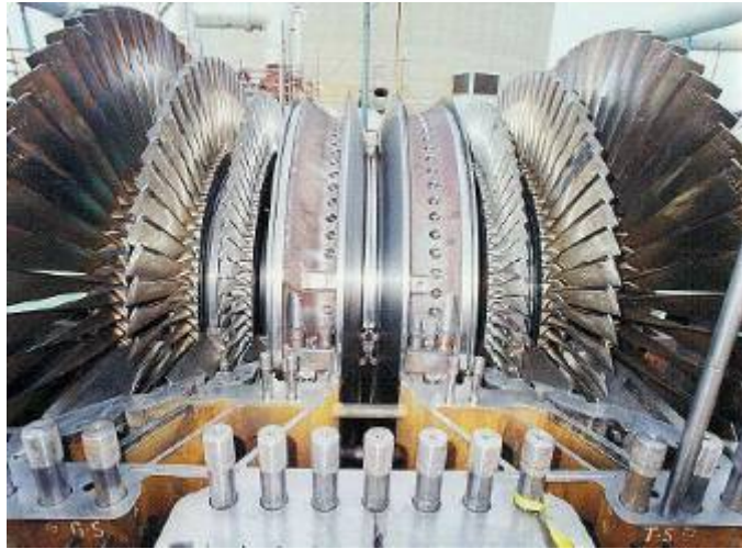
Figure 5 – Salem 1 LP Turbine with Rotor and 1 st upper blade ring installed
