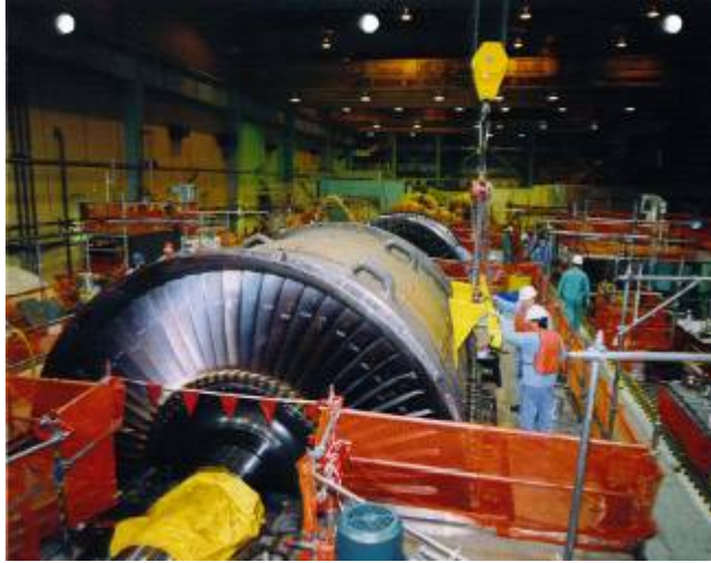
Figure 6 – LP Turbine Installation at SSES
