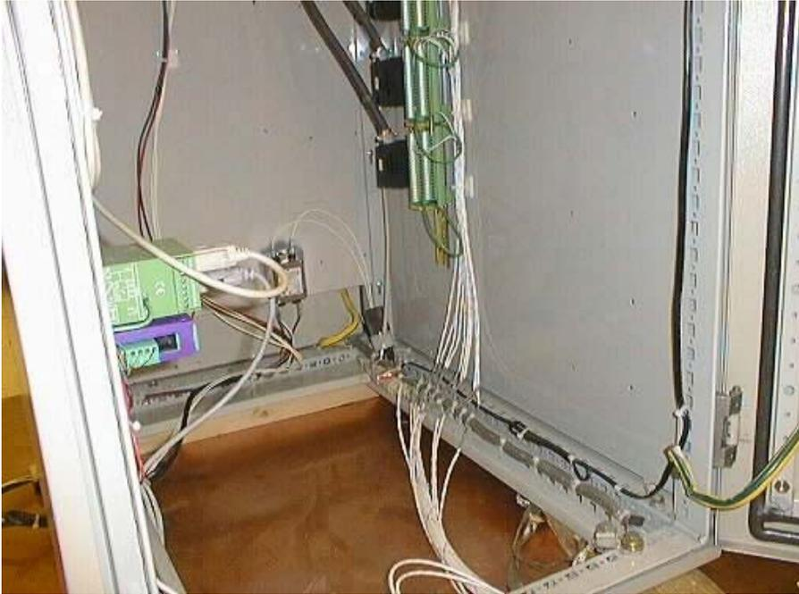
Figure 9-5—Bottom Cable Entry Area
