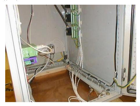
Figure 14-9. Bottom Cable Entry Area
