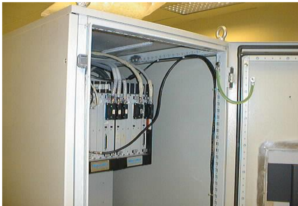
Figure 14-8. Door Bonding
