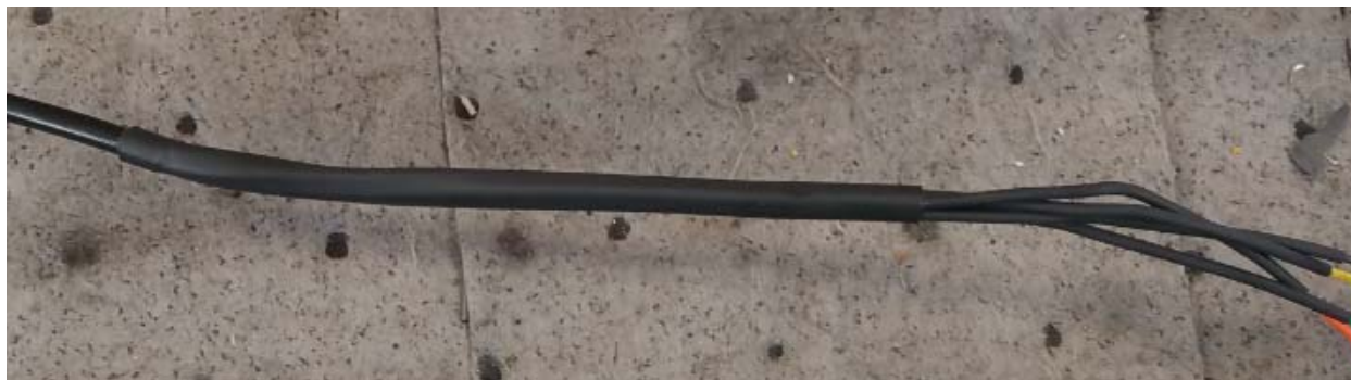
Figure 10. Large Heat Shrink Tubing Installed
