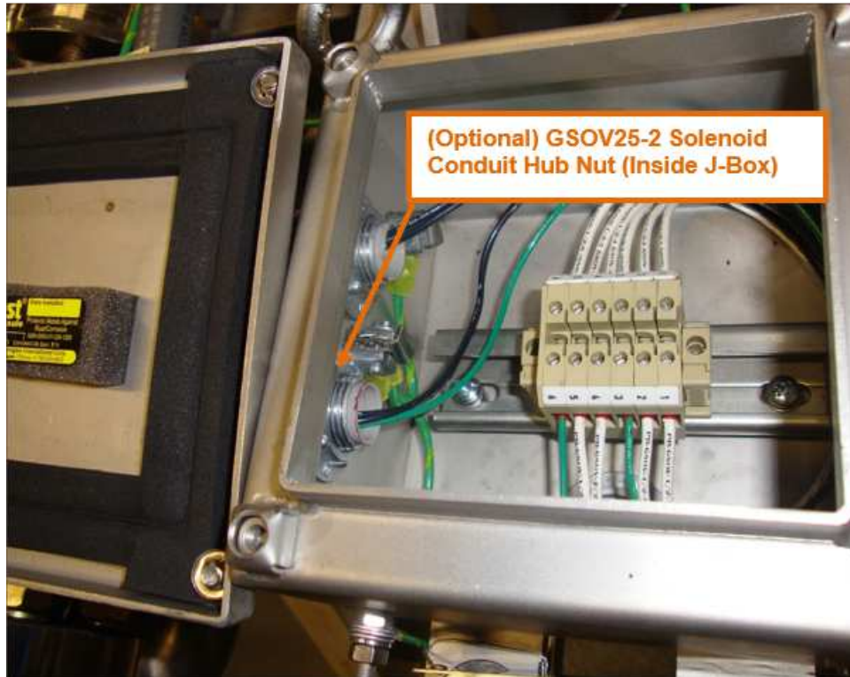
Figure 2-8. GSOV25-2 Solenoid Conduit Removal
