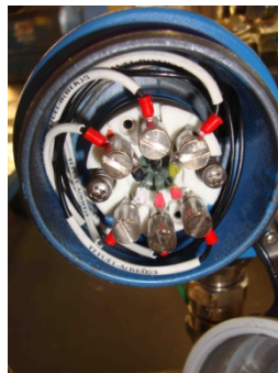
Figure 2-2. Dual Element RTD Terminal Block Connections
