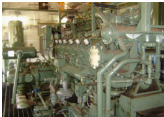
Waukesha 7044 engine driving a gas compressor
