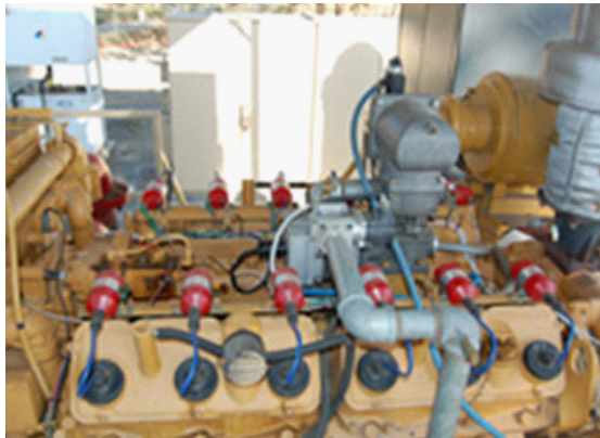
Caterpillar 3412 engine driving a water pump
