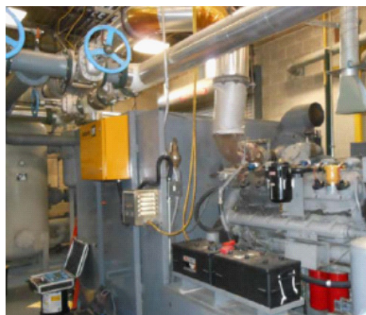
Caterpillar 3412 engine driving an air compressor
