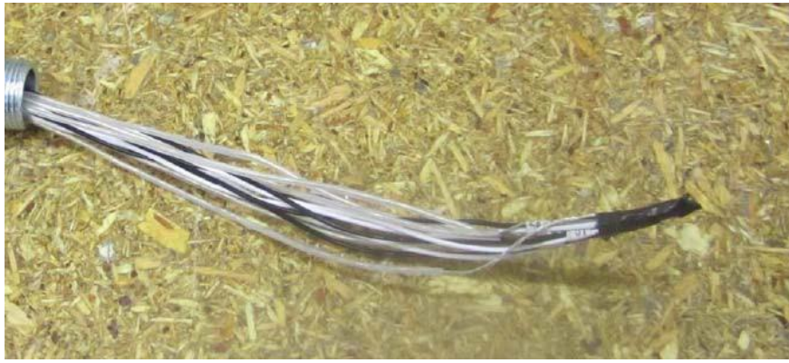
Figure 3-7. Running Cable through Conduit
