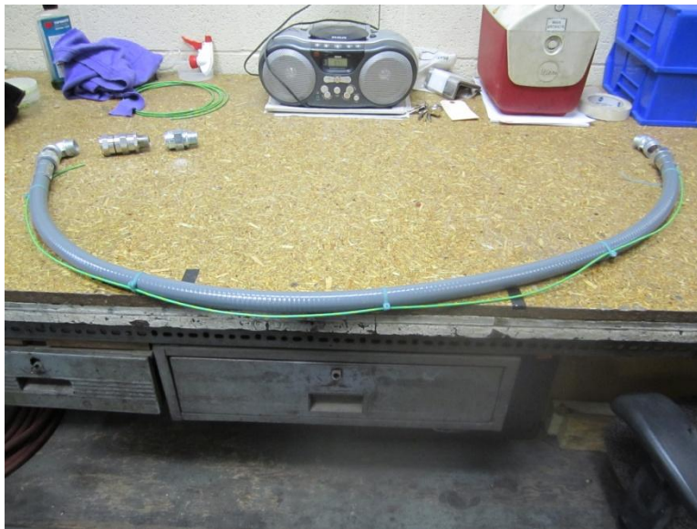
Figure 3-6. Tefzel Grounding Wiring Installation
