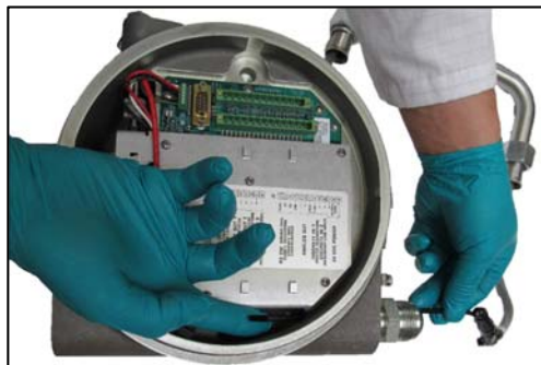
F. CPC cable installation
