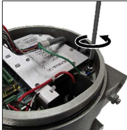
Figure 4-8. CPC-II Ground wire unscrewing.
